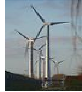
Wind power plant
