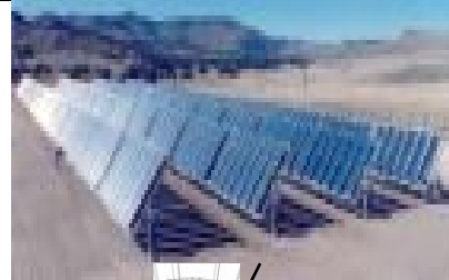
Photovoltaics power plant
