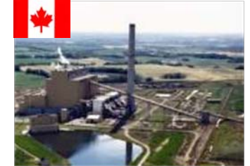
Transalta Canada - >200 MWe Chilled Ammonia - Coal
