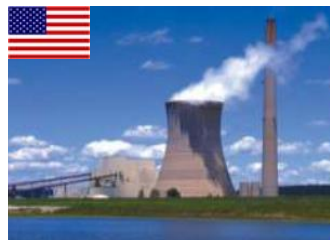
AEP Mountaineer USA - 235MWe
