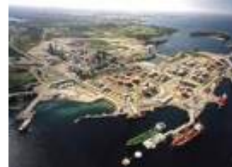
Statoil Mongstad Norway - 40 MWth Chilled Ammonia - Gas
