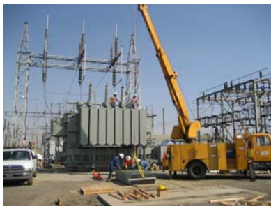
SMUD crew rehabilitating a transformer during a planned outage.
