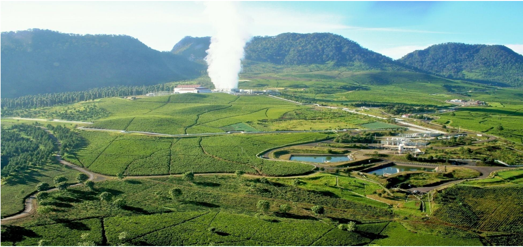
Wayang Windu Geothermal Power Station – West Java
