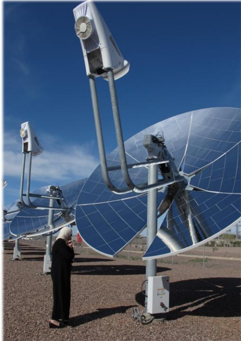
Maha Al-Ramahi, Interconnection of the Grid Section Head at NEPCO, inspects the reflective mirrors on a 3kW concentrated solar power (CSP) Stirling Dish-Engine. 40% of the electricity needs at the Frito Lay facility in Casa Grande, AZ are met by solar PV and CSP.
