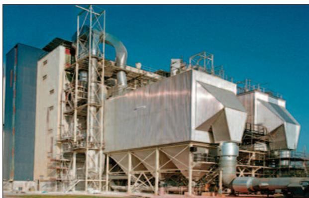
**Figure 2** ESP photo (FLSmith, 2012a)
