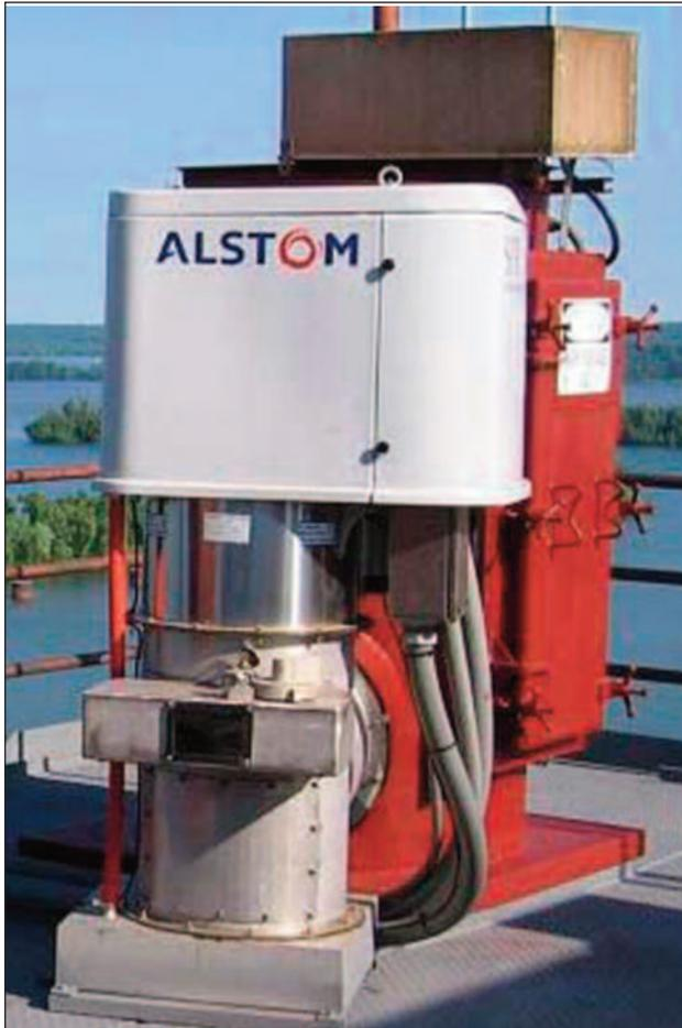
**Figure 5 Switched integrated rectifier photo**
