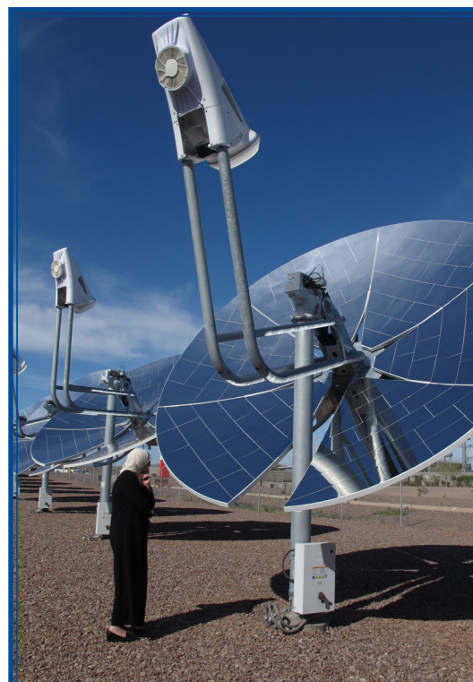
NEPCO's Eng. Maha Al-Ramahi inspects a concentrated solar satellite during a site visit to an APS customer facility.
