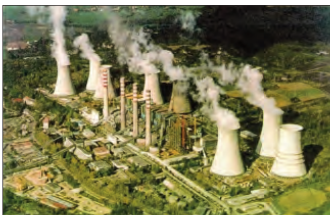
Figure 12 Turów power plant, Poland (photograph courtesy of Elektrownia Turów SA)
