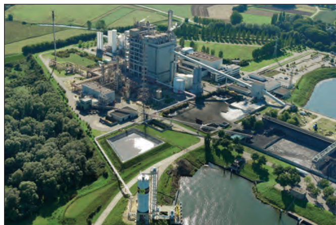
Figure 10 The Willem Alexander IGCC plant at Buggenum in The Netherlands (photograph courtesy of NUON)
