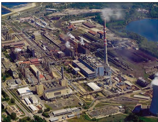
Figure 5 The Vresova IGCC plant in the Czech Republic (photograph courtesy of Sokolovska uhelná)
