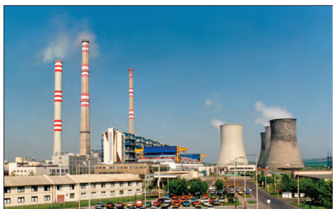
Figure 4 Part of the Pocerady power plant site in the Czech Republic (photograph courtesy of ČEZ)
