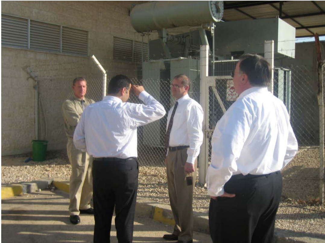
Mike Rudek, SMUD; Fouad Dagher, National Grid and Lawrence Reilly visit a 33 kv substation near the Dead Sea.
